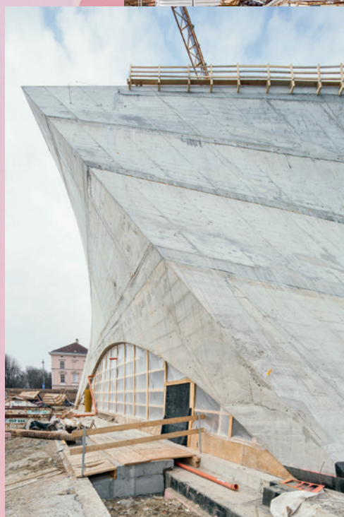
Rohbau der Landesgalerie NOE, April 2018 © LOXPix
